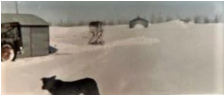
Access to shop and the fuel tank completed.
